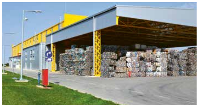
Our recycling plant in Serbia.
