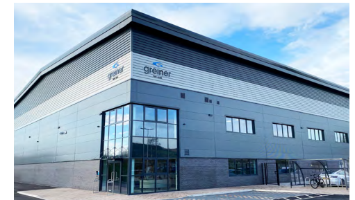
New warehouses and office buildings for Greiner Bio-One UK
